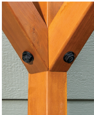
Structural wood screw and hex-head washer
